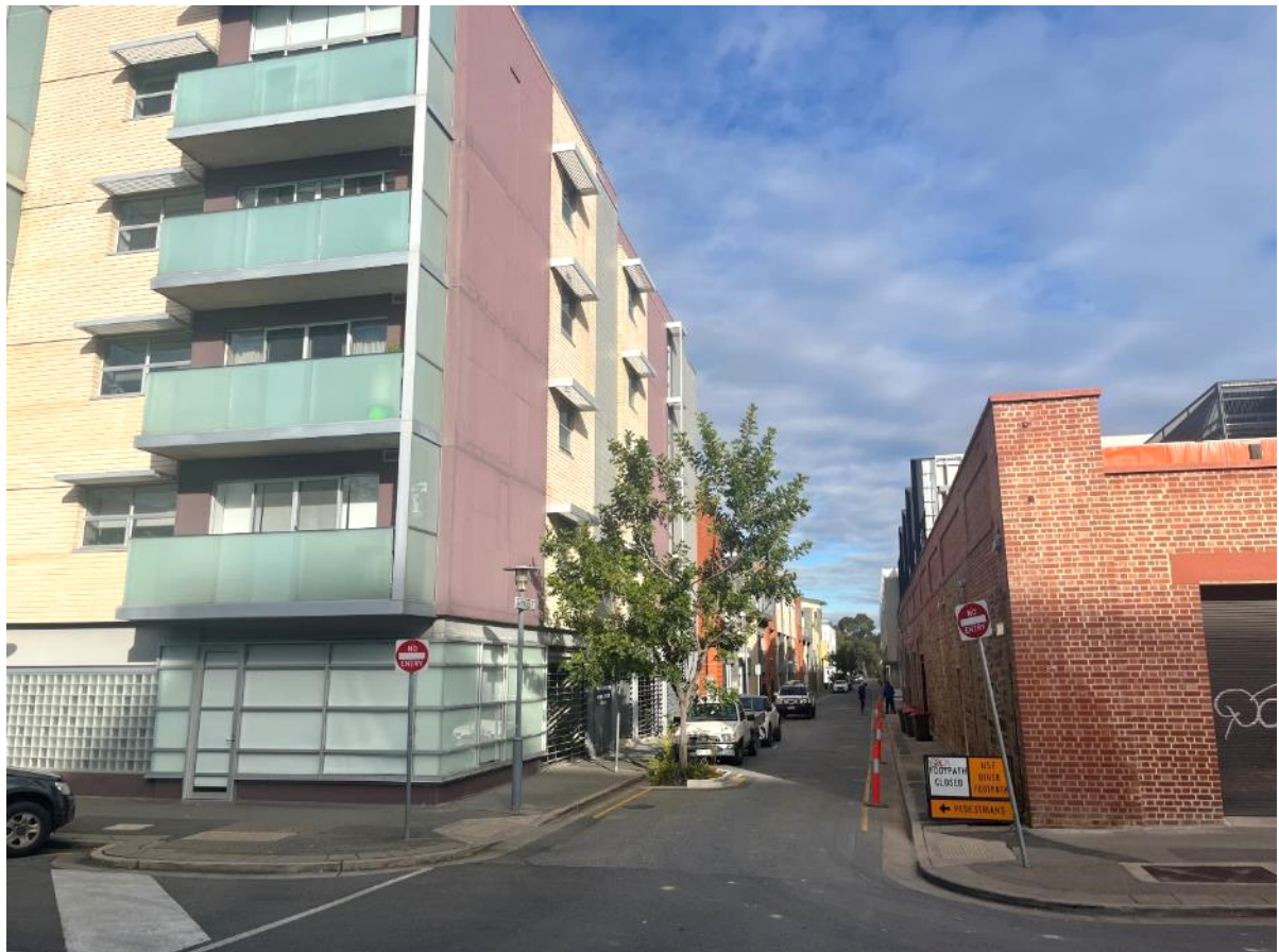
Photo 3.2 – view of subject site and adjacent residential flat building looking south
