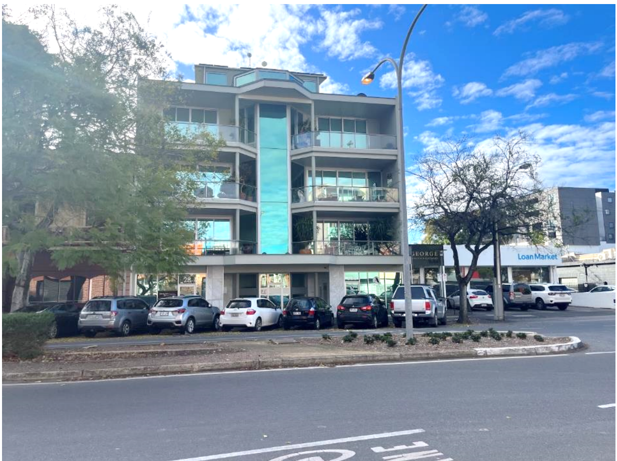
Photo 3.8 – mixed use building opposite the subject site at 28-30 Halifax Street
