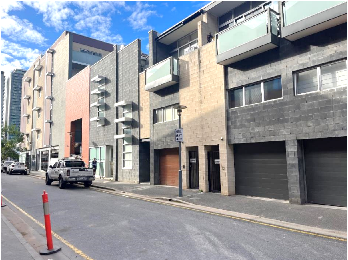
Photo 3.7 – view of dwellings on eastern side of Symonds Place
