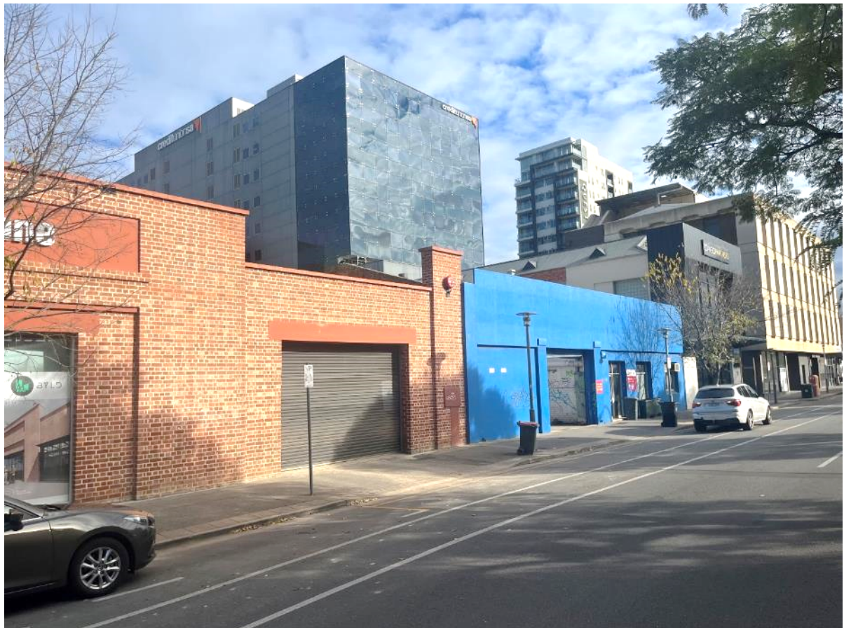
Photo 3.6 – view of subject site and adjacent carpark building looking southwest
